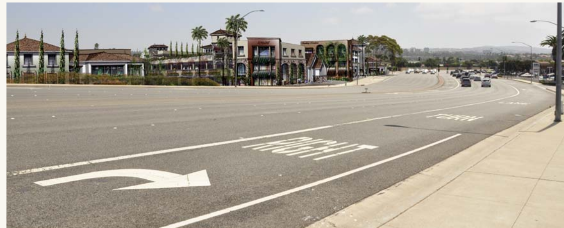
View from Bridge along East Coast Highway
